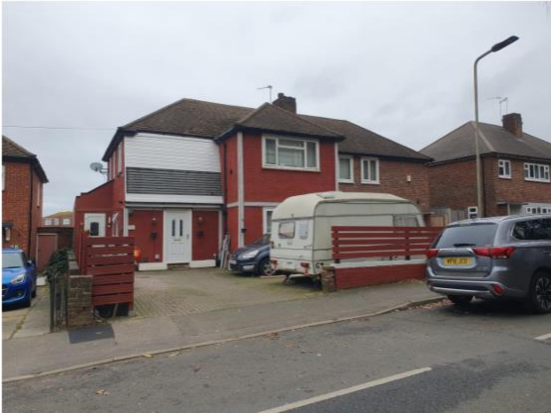
Figure 6: Photograph of the site from the front:
